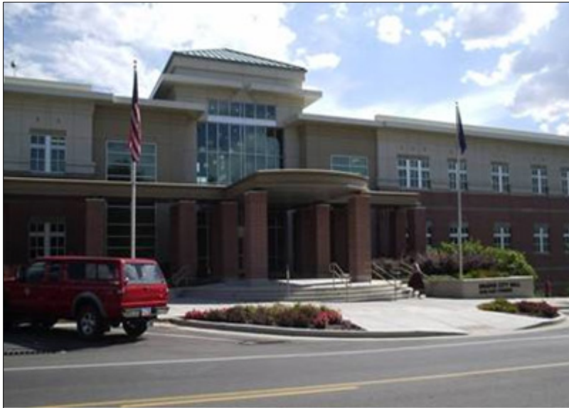
Draper City Hall on Pioneer Road (12400 South)
