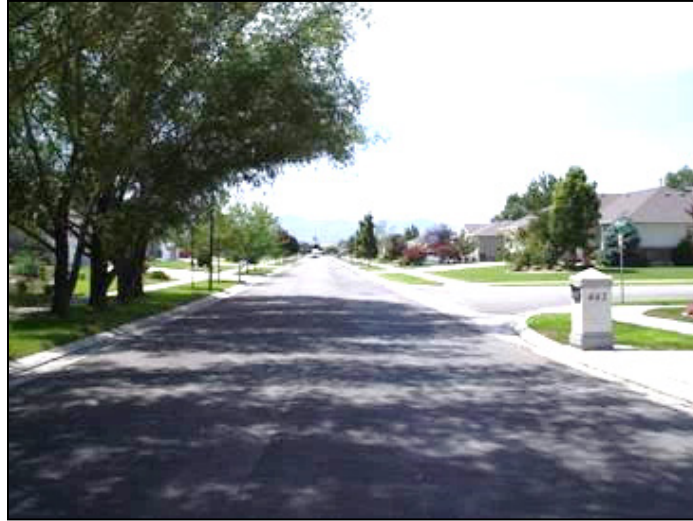
Typical Residential Street in Draper City
