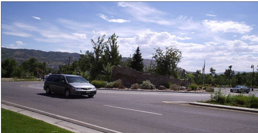
1300 East, Pioneer Road (12400 South) Roundabout
