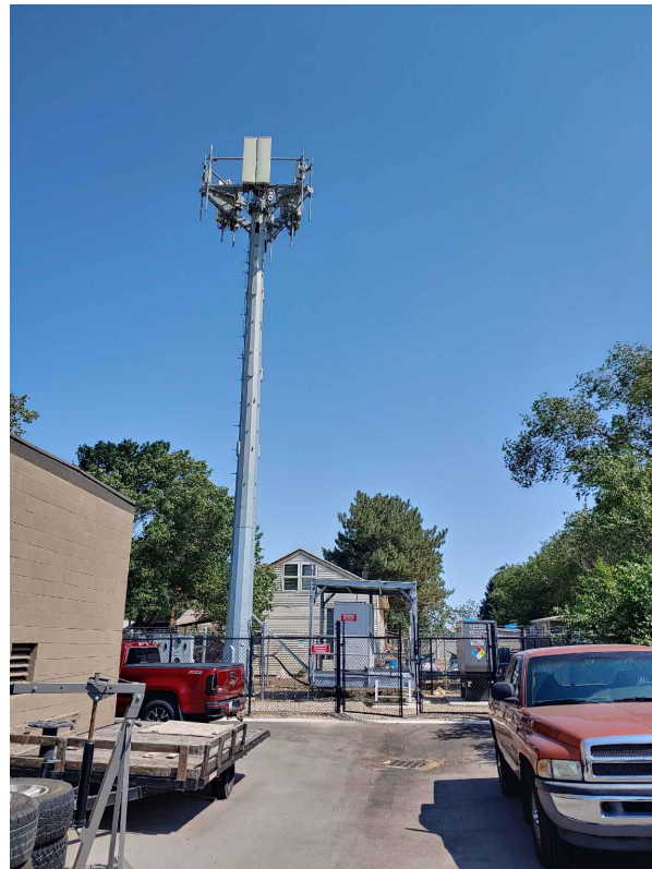
VIEW OF EXISTING SITE ELEVATION
