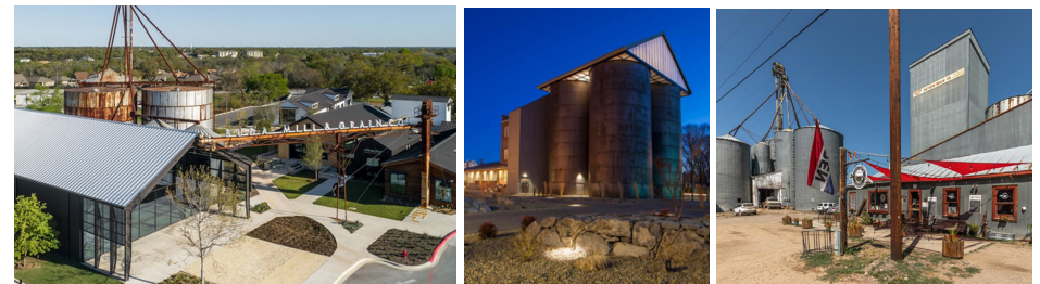
Adaptive reuse examples of silos and mills from around the United States.
